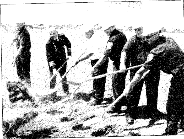
Ground breaking for the new Frederick Firestone Fire Protection District Fire Station #3
